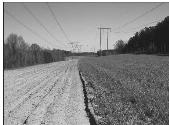
Keeping rights-of-way clear of vegetation and brush helps to keep BCREMC's power system reliable and reduces the risk of power outages.
